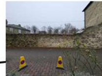
View 1 - Site photograph (2025) Showing new yellow brick infill in the brick boundary wall to Willow Walk (c. 2000)
