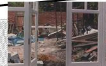
View 2 - Site photograph (c. 2000) Conservatory being built in the background
